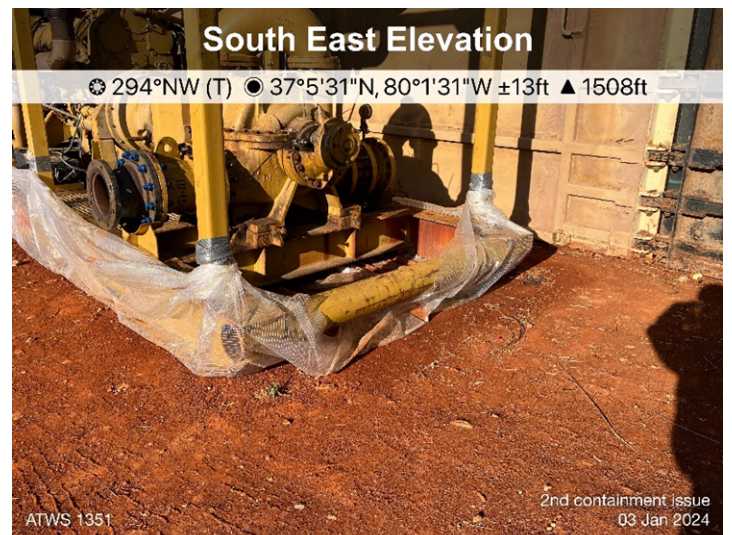
Figure 4: ATWS 1351, 2 nd containment require repair and reinstall per the spec.
