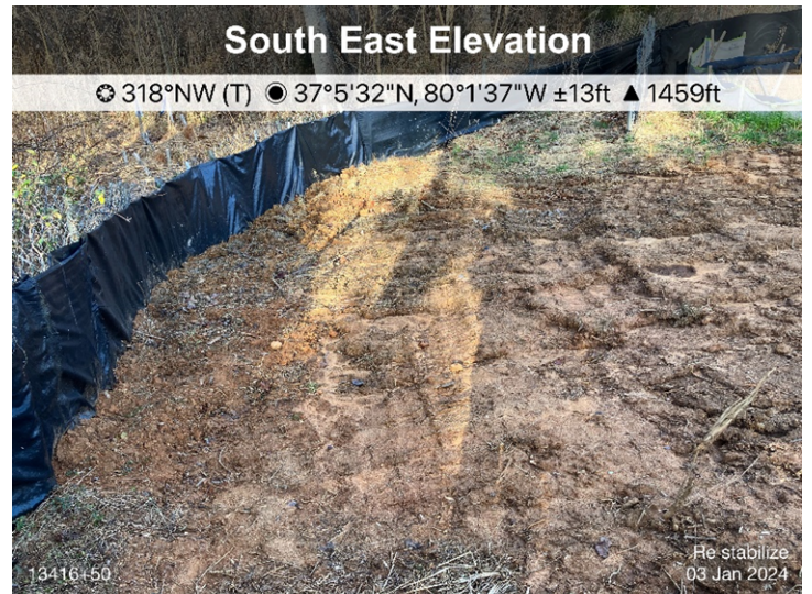
Figure 2: Sta 13416+50, re stabilize denuded area.
