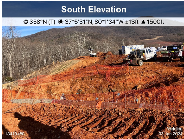
Figure 1: Sta 13419+80, ECD's are in place.
