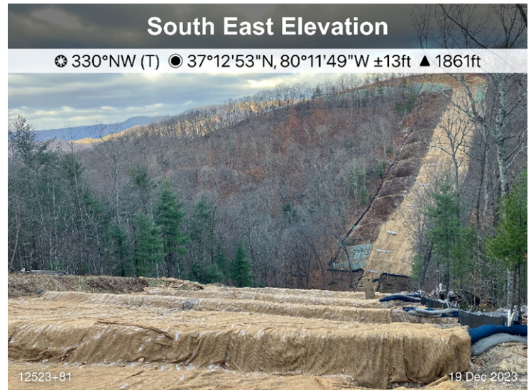
Figure 2: Sta 12523+81, ECD's and stabilization are in place.
