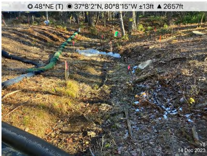
Figure 3: Stream S-Y8 – Controls installed and functioning properly.
