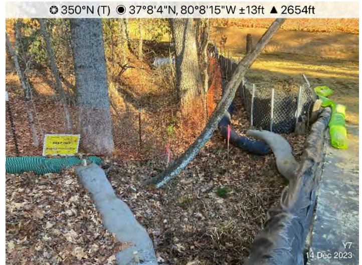
Figure 4: ATWS 1306 – Dewatering structure installed and functioning properly.
