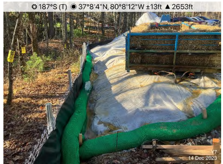
Figure 4: ATWS 1306 – Dewatering structure installed and functioning properly.
