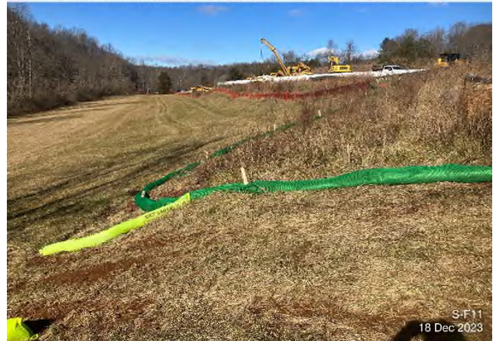
Figure 4: ATWS 351A – Controls installed and functioning properly.
