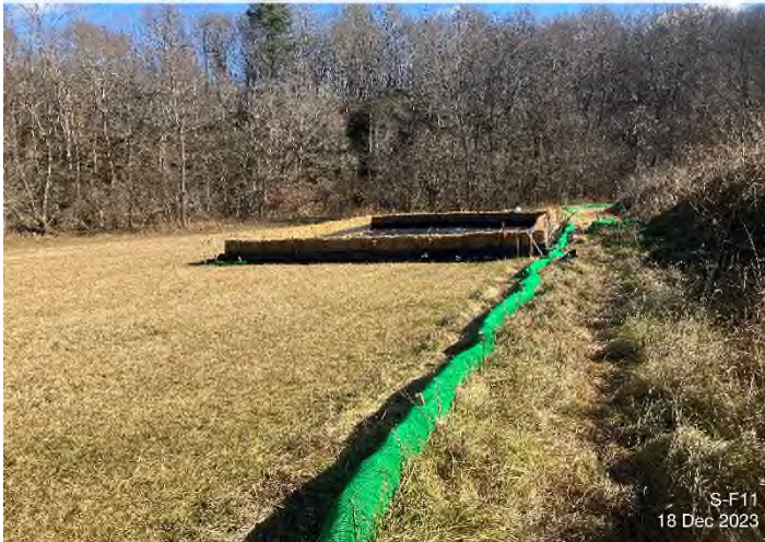
Figure 3: ATWS 351 – Controls installed and functioning properly.
