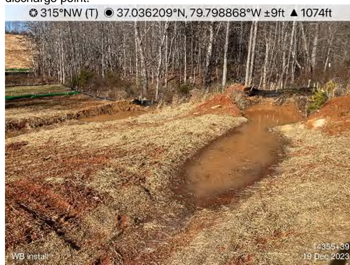
Figure 2: STA 14355+39 – Waterbar lower than end treatment discharge point.
