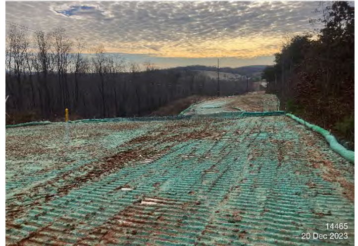
Figure 4: STA 14524+00 – Controls installed and functioning properly.
