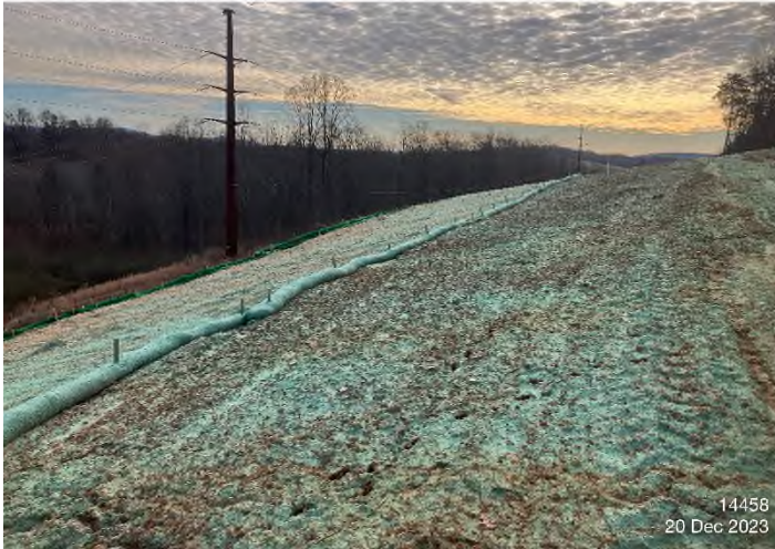
Figure 3: Stream S-G20 – Controls installed and functioning properly.
