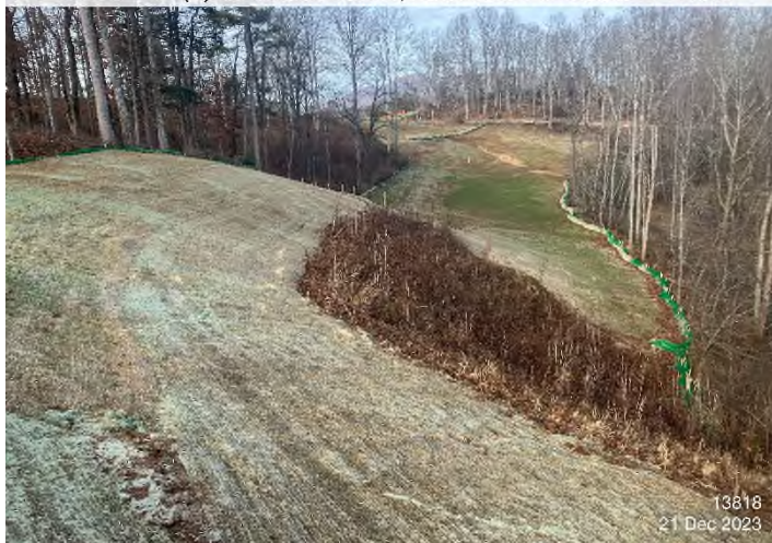
Figure 3: Stream S-CD6 – Controls installed and functioning properly.
