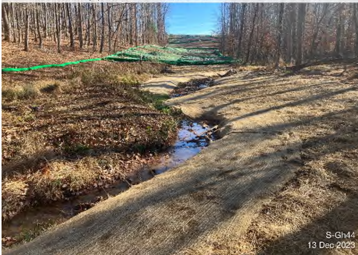
Figure 3: Stream S-GH44 – Controls installed and functioning properly.
