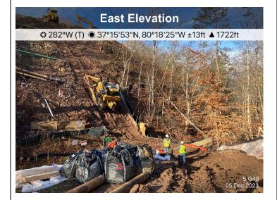
Figure 2: Designated crossing S-G38, ECD's and stabilization are in place.
