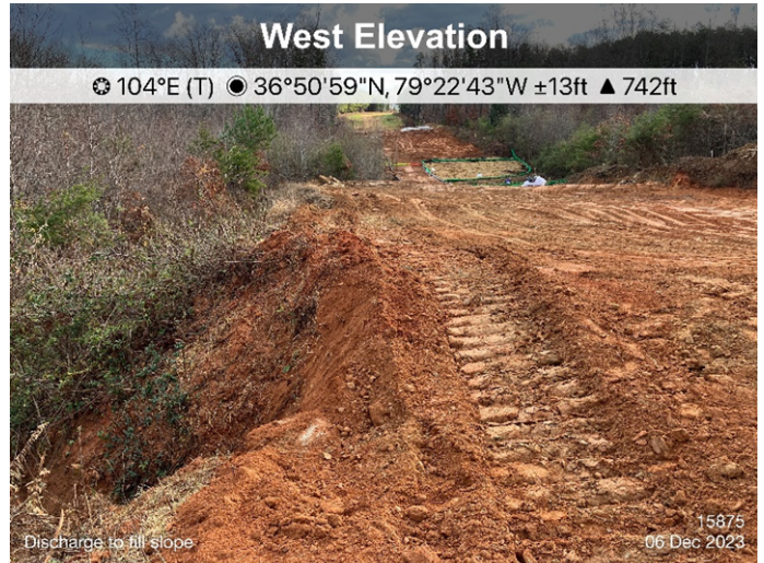
Figure 2: Sta 15875, discharge to fill slope.
