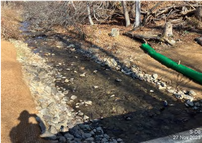
Figure 3: Stream S-D8 – Controls installed and functioning properly.
