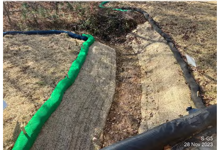
Figure 4: Stream S-G5 – Controls installed and functioning properly.
