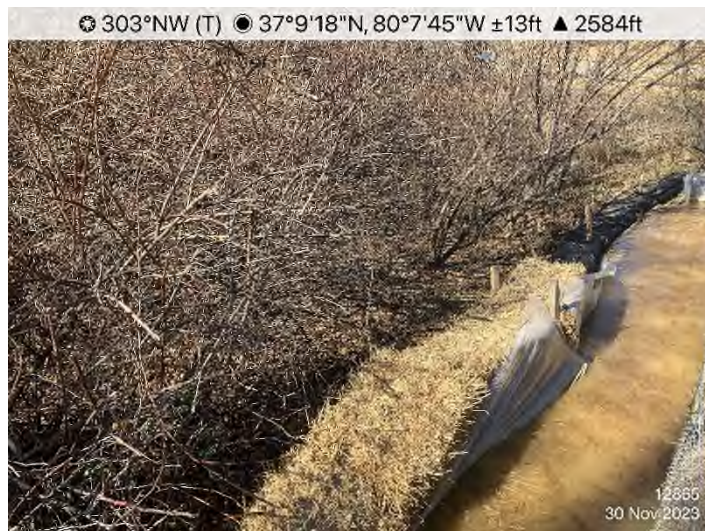
Figure 3: STA 12865+00 – Discharge point of dewatering structure on west side of Bottom Creek Road. Discharging to well vegetated area as sheet flow.
