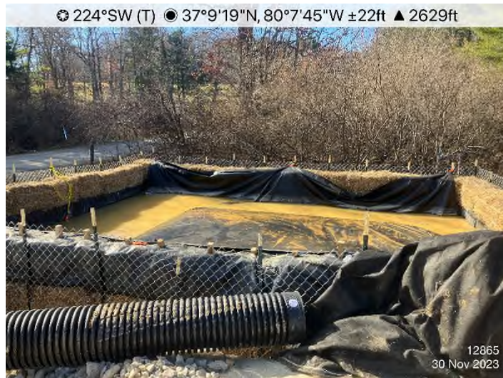
Figure 3: STA 12865+00 – Discharge point of dewatering structure on west side of Bottom Creek Road. Discharging to well vegetated area as sheet flow.
