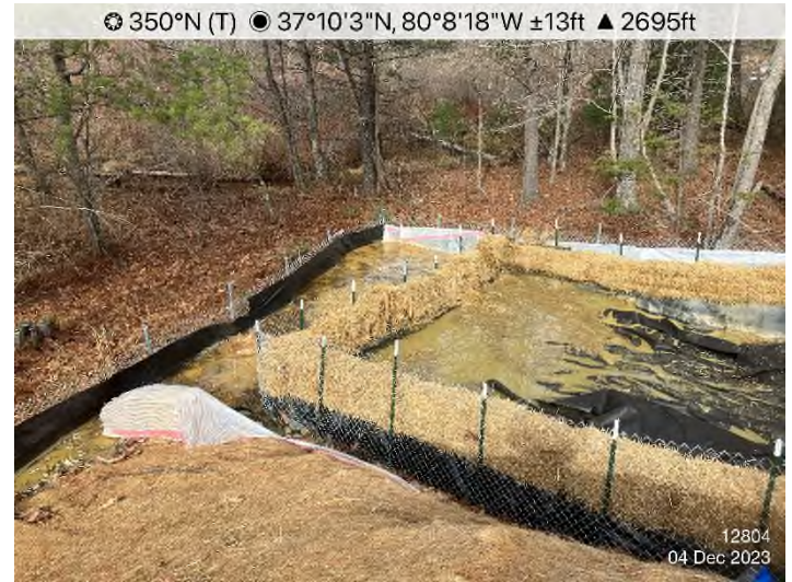
Figure 2: STA 12804+00 – Dewatering structure maintenance needed. Remove sediment from within dewatering structure.
