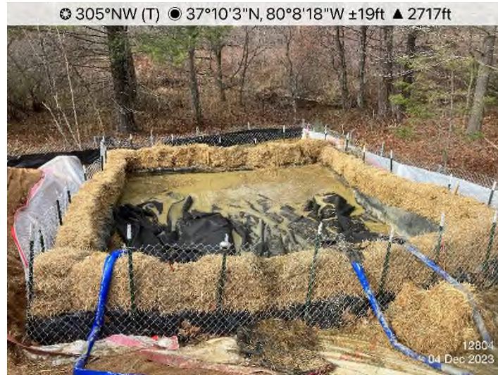
Figure 1: STA 12804+00 – Dewatering structure maintenance needed. Remove sediment from within dewatering structure.
