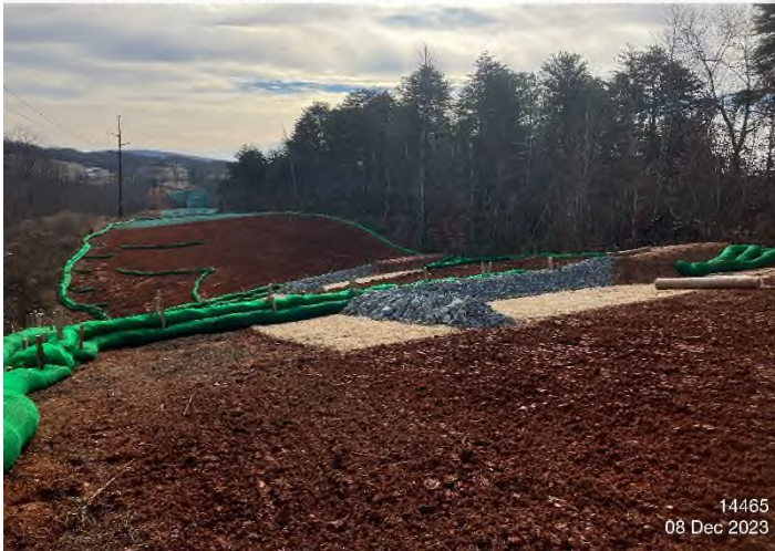
Figure 3: STA 14465+00 – Controls installed and functioning properly.
