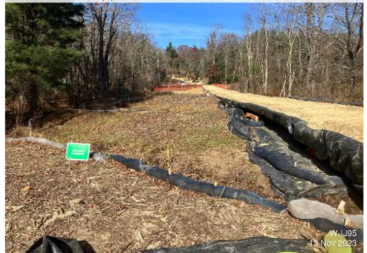
Figure 4: Wetland W-IJ95 – Controls in place and functioning properly.
