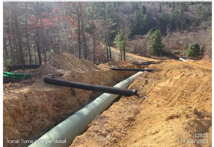
Figure 4: STA 12929+00 to 12937+00 – Install trench pipes per specification.
