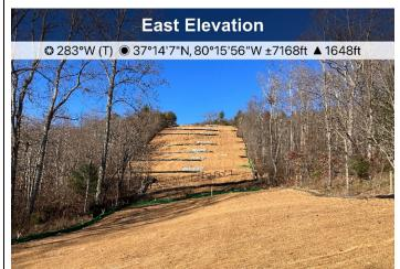
Figure 3: Designated crossing S-C29, ECD's are in place.
