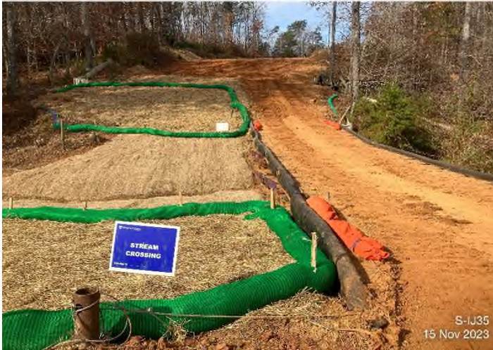
Figure 1: Stream S-IJ35 – Controls in place and functioning properly.
