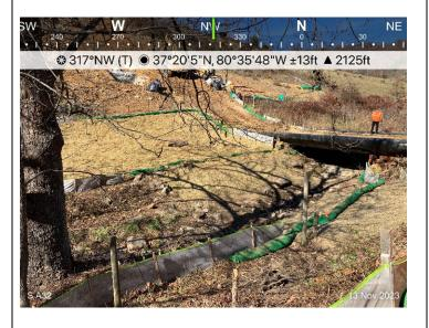
Figure 2: Designated crossings S-Z9, ECD's are in place for active construction.
