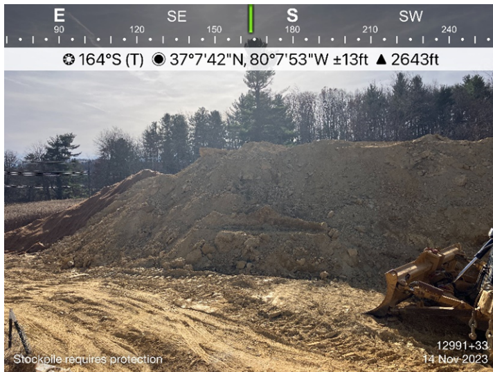
Figure 3: Sta 12991+33 stockpile requires re stabilization.
