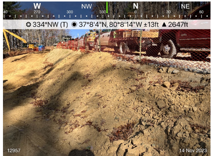
Figure 2: Sta 12957 fill slope requires re stabilization.
