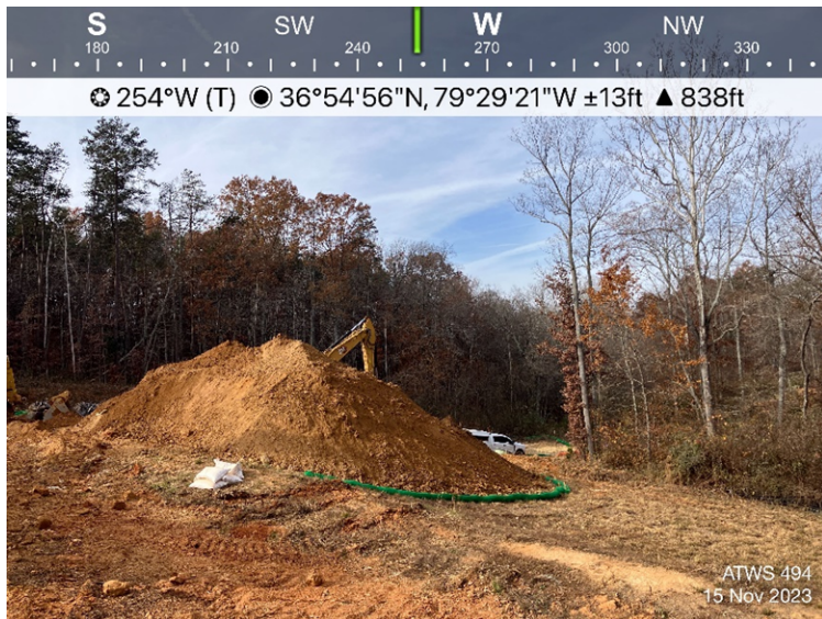
Figure 3: ATWS 494, ECD's are in place.
