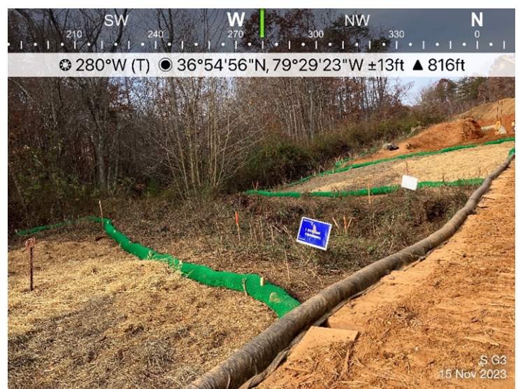
Figure 4: Designated crossing S-G3, ECD's are in place.
