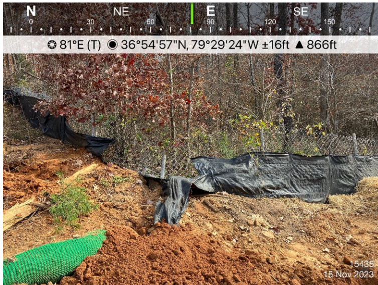
Figure 1: Sta 15435 SSF requires repair.
