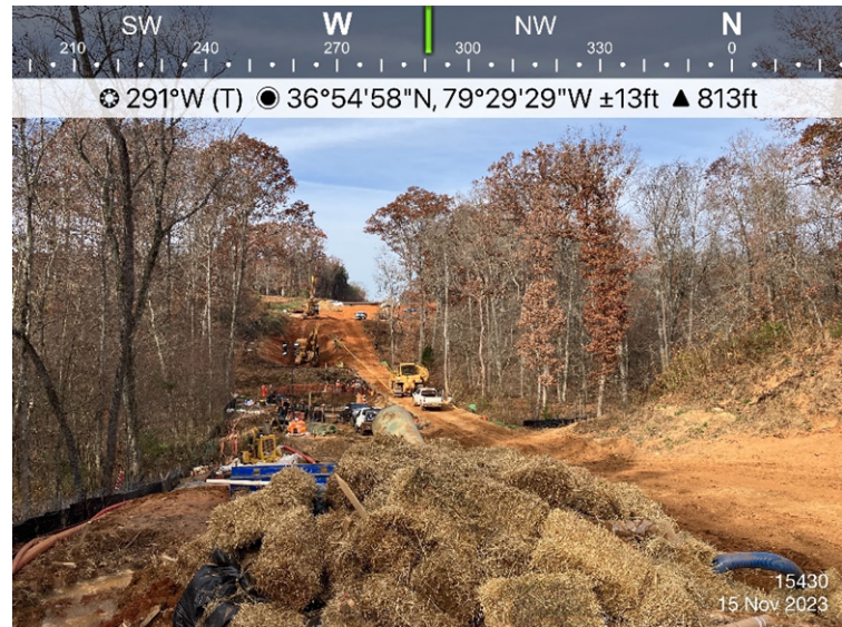
Figure 2: Sta 15430 ECD's are in place.
