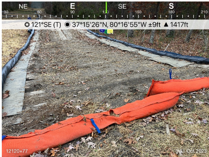
Figure 1: Sta 12120+77 CFS wattle torn and requires repair.
