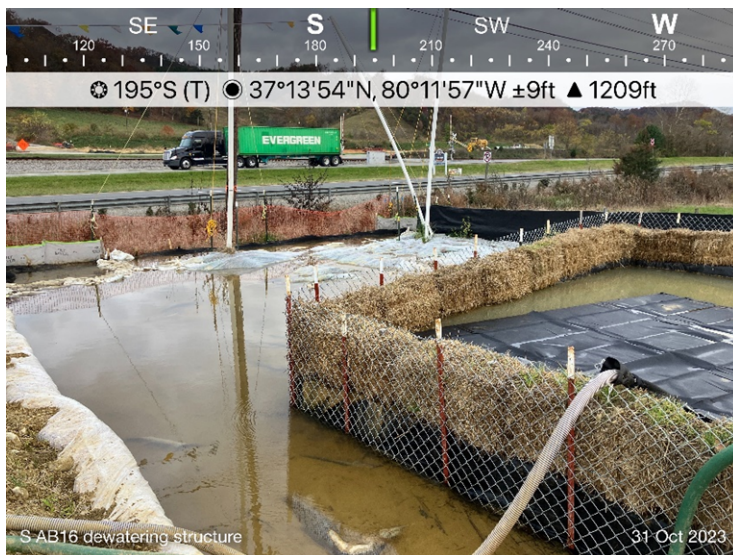
Figure 3: Dewatering structure for designated crossing S-AB16.
