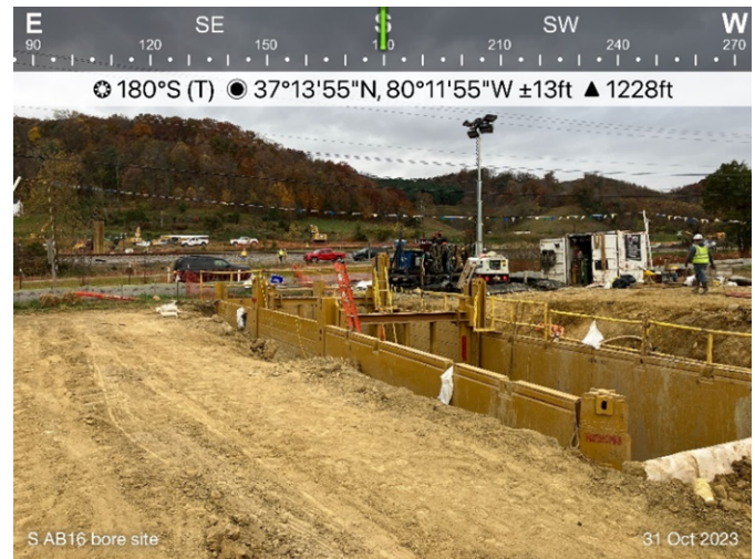
Figure 2: Bore site for designated crossing S-AB16, ESC's are in place.
