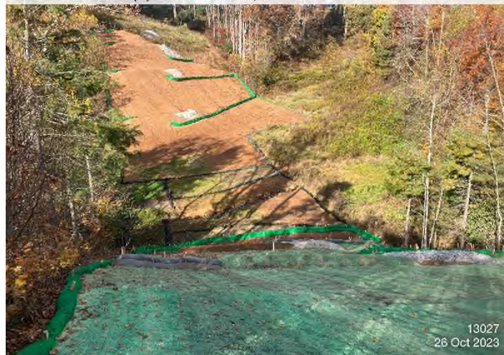
Figure 4: STA 13353+00 – Controls installed and properly functioning.
