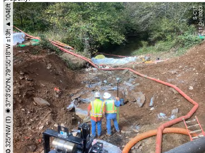
Figure 4: Stream S-C14 – Controls in place and functioning properly.
