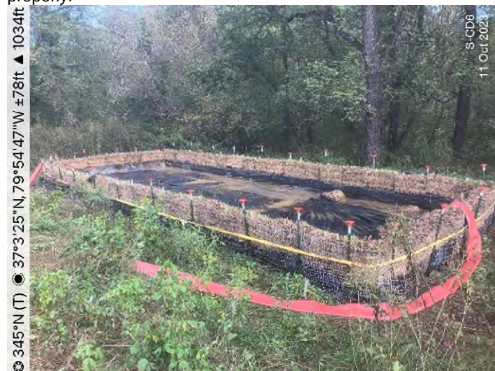
Figure 1: Stream S-CD6 – Controls in place and functioning properly.
