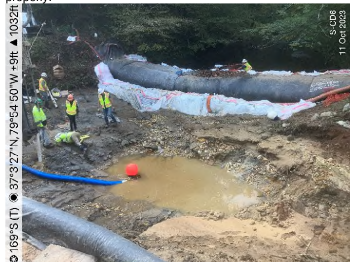
Figure 2: Stream S-CD6 – Controls in place and functioning properly.
