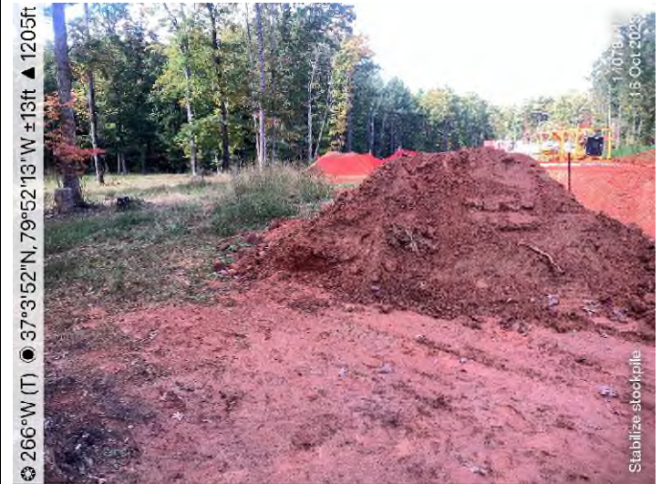
Figure 4: STA 14079+00 – Install additional perimeter controls to prevent sediment from leaving ROW.
