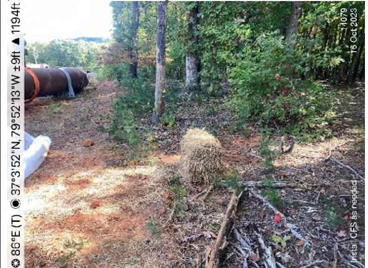
Figure 4: STA 14079+00 – Install additional perimeter controls to prevent sediment from leaving ROW.
