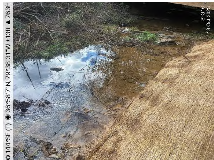
Figure 3: Stream S-G16 – Erosion matting, and seed applied to stabilize repaired bank. Controls repaired and reinstalled.
