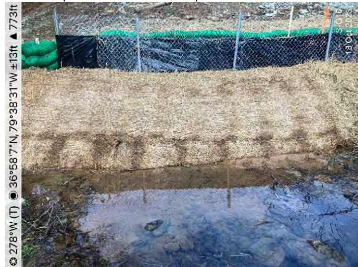
Figure 3: Stream S-G16 – Erosion matting, and seed applied to stabilize repaired bank. Controls repaired and reinstalled.
