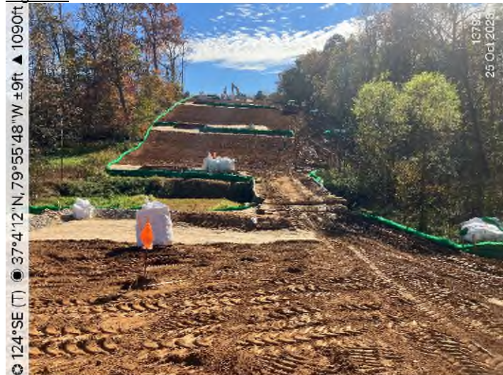
Figure 3: STA 13792+00 – Final restoration controls installed.
