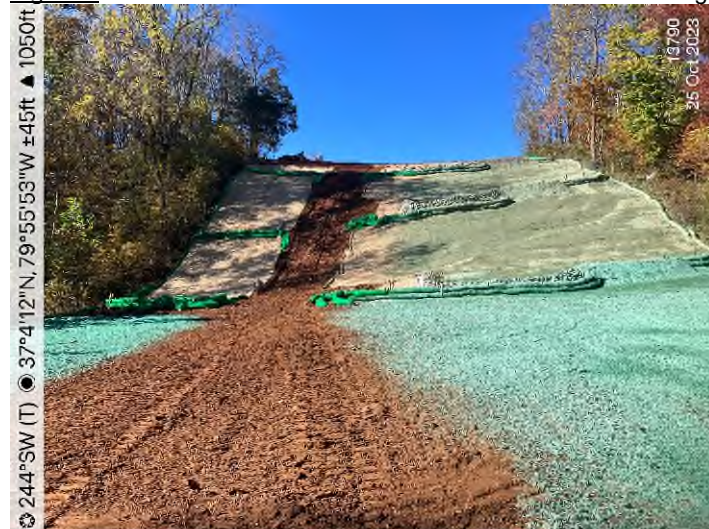
Figure 4: STA 13790+00 – Final restoration controls and seeding.
