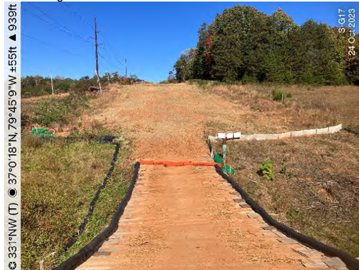
Figure 3: Stream S-G17 – Controls installed and properly functioning.
