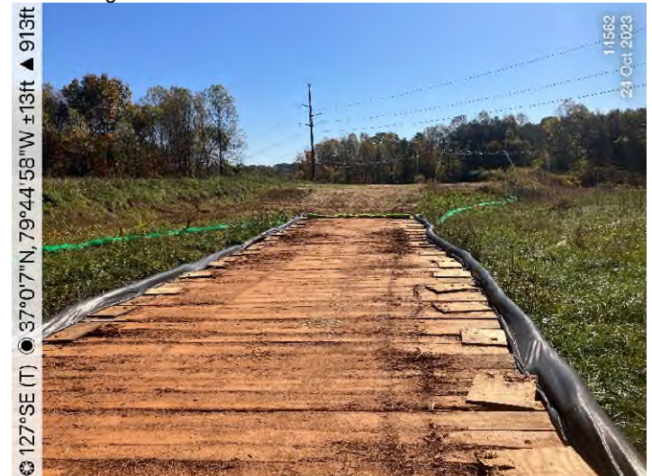
Figure 4: STA 14562+00 – Controls installed and properly functioning.
