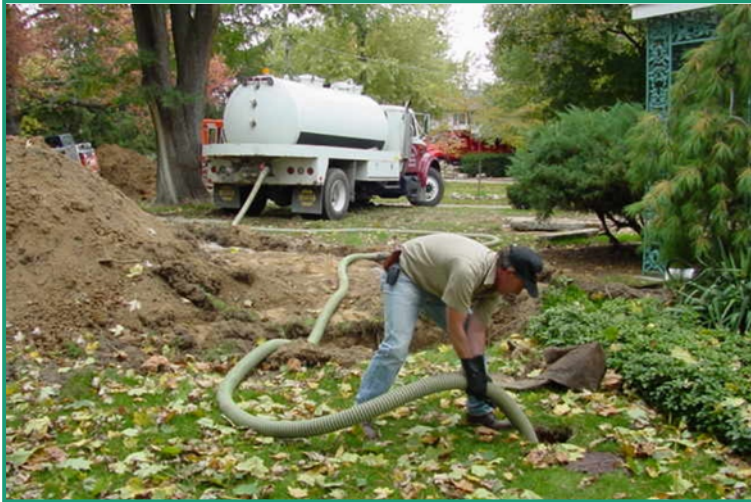
Septic System Pump out
