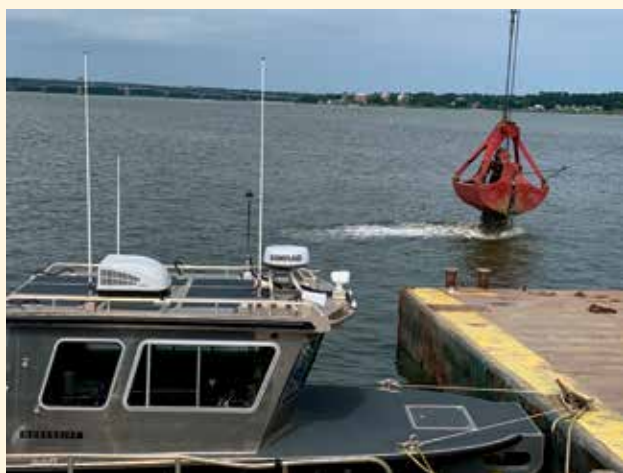
Crushed granite being placed at the site of oyster reef restoration in the York River. The granite will form the hard substrate on which oyster spat will settle and ultimately form a 3-D reef. Photo by Andrew Button, VMRC.
