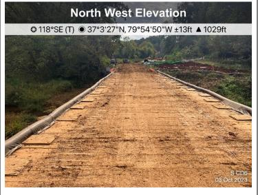
Figure 4: Sta 13997+79 near designated crossing S-C36, ESC is in place.
