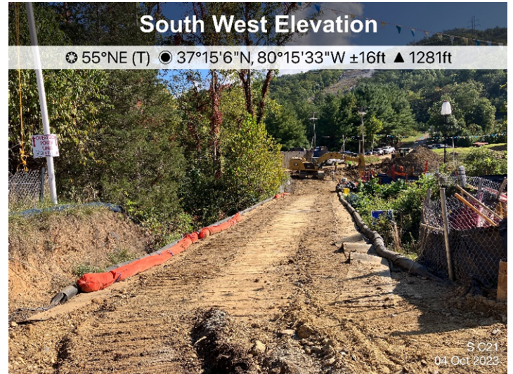
Figure 4: Designated crossing S-0011, ECD's are in place.
