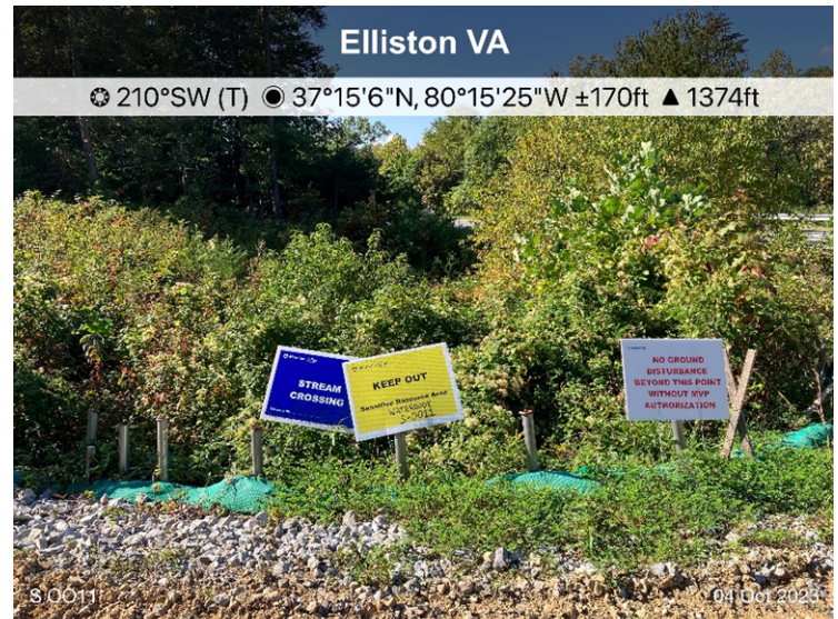
Figure 4: Designated crossing S-0011, ECD's are in place.
