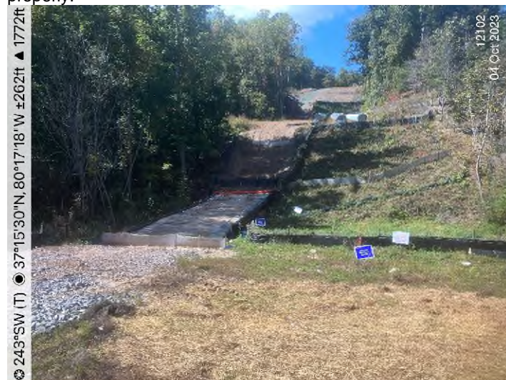
Figure 4: STA 12102+00 – Controls in place and functioning properly.
