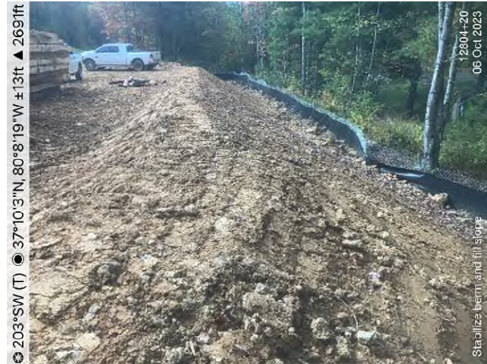
Figure 1: STA 12804+20 to 12806+20 – Stabilize fill slopes and diversion berms.
