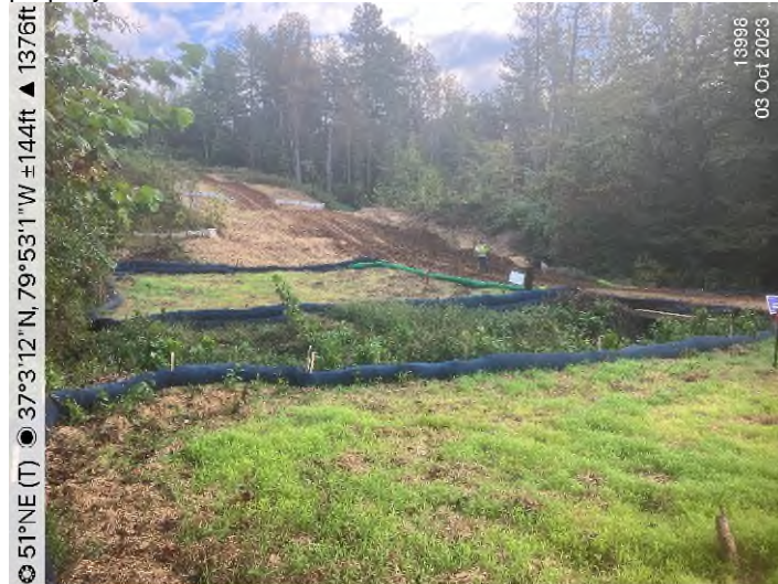
Figure 1: STA 13998+70 – Controls in place and functioning properly.
