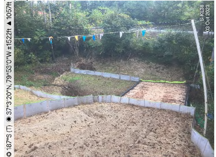
Figure 2: Stream S-KL38 – Controls in place and functioning properly.
