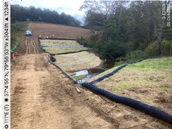
Figure 1: Stream S-E28(3) – Controls in place and functioning properly.
