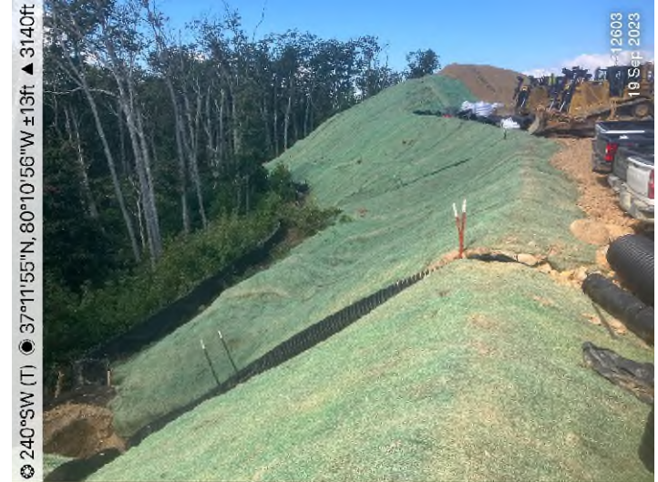
Figure 2: STA 12603+00 – Controls in place and functioning properly.
