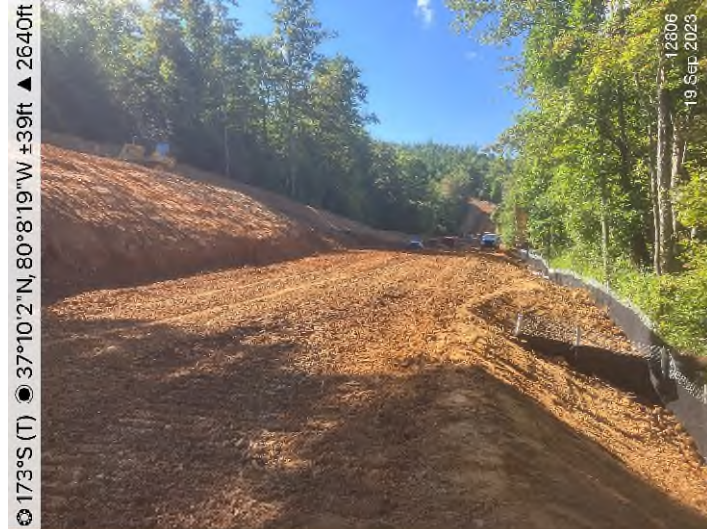
Figure 1: STA 12806+00 – Controls in place and functioning properly.
