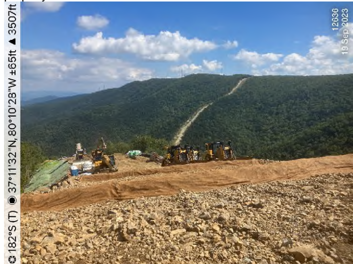
Figure 3: STA 12636+00 – Controls in place and functioning properly.
