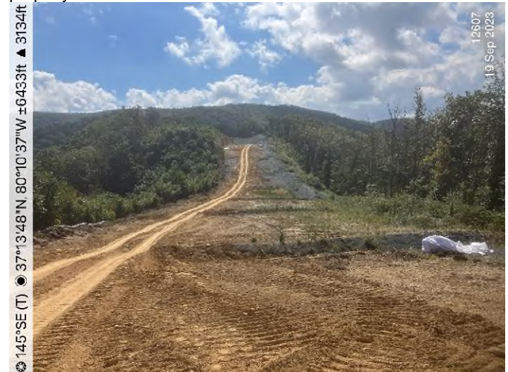
Figure 4: STA 12607+00 – Controls in place and functioning properly.
