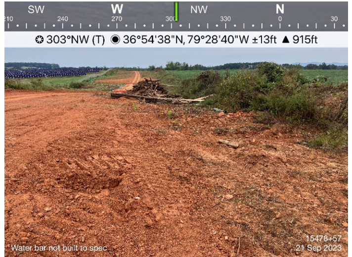
Figure 2: Sta 15478+57 waterbar does not extend to sump.
