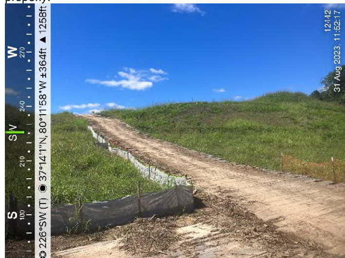
Figure 2: STA 12442+00 – Controls in place and functioning properly.
