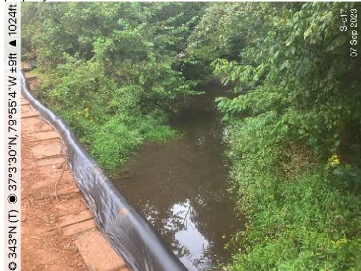
Figure 3: Stream S-C17 – Controls in place and functioning properly.
