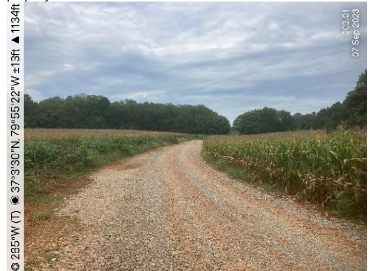
Figure 4: MVP-FR-303.01 – Controls in place and functioning properly.
