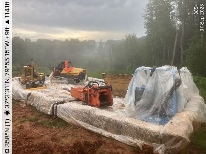
Figure 1: STA 13854+00 – Controls in place and functioning properly.
