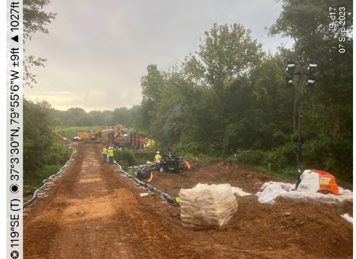
Figure 2: STA 13862+00 – Controls in place and functioning properly.
