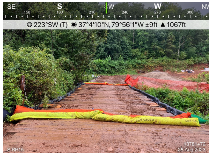
Figure 4: Designated crossing S-RR15, ECD's are in place.
