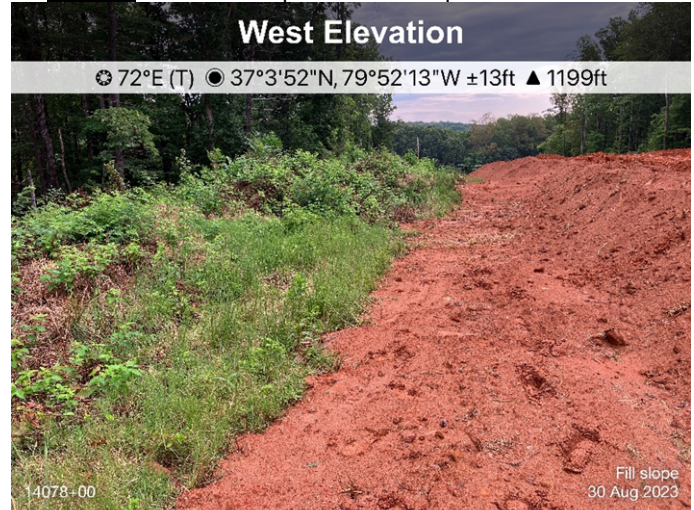
Figure 6: 14078 fill slope not built to spec.
