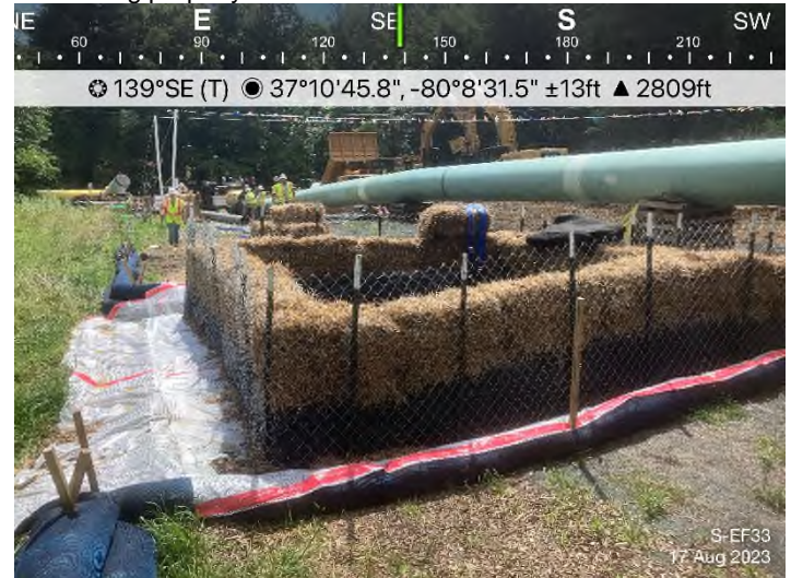
Figure 4: Stream S-EF33 – Dewatering structure in place and functioning properly.
