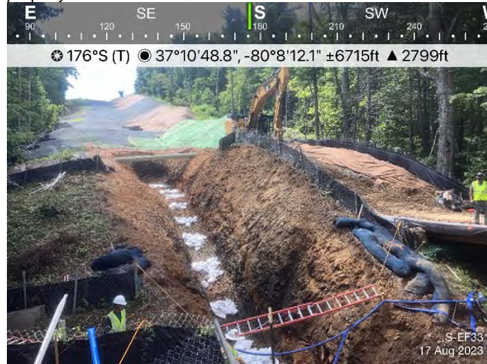
Figure 3: Stream S-EF33 – Controls in place and functioning properly.
