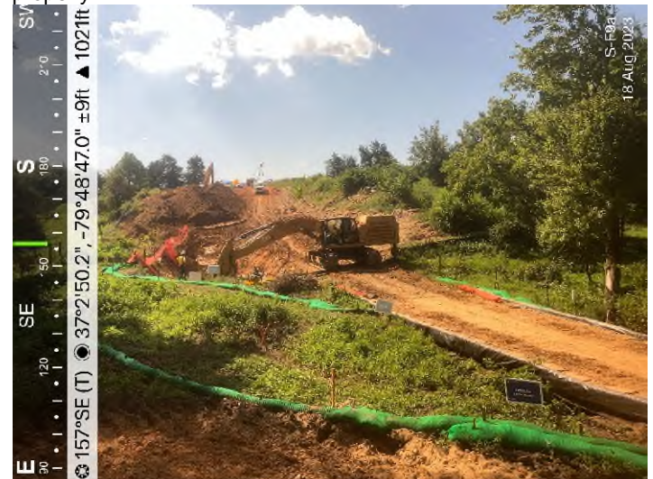
Figure 4: Stream S-F9a – Controls in place and functioning properly.
