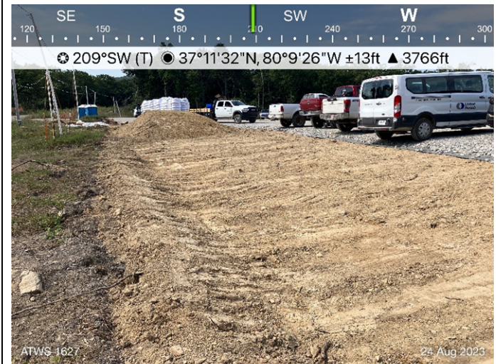
Figure 4: ATWS 1627, denuded area requires stabilization.
