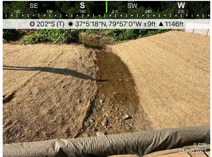
Figure 2: Designated crossing S-E29, ECD's are in place.
