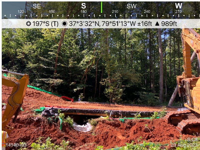
Figure 3: Designated crossing S-C8, ECD's are in place.
