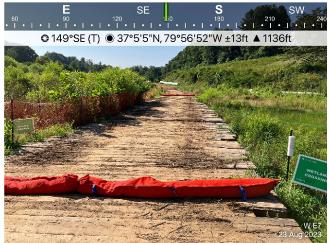
Figure 4: Designated crossing W-E7, ECD's are in place.
