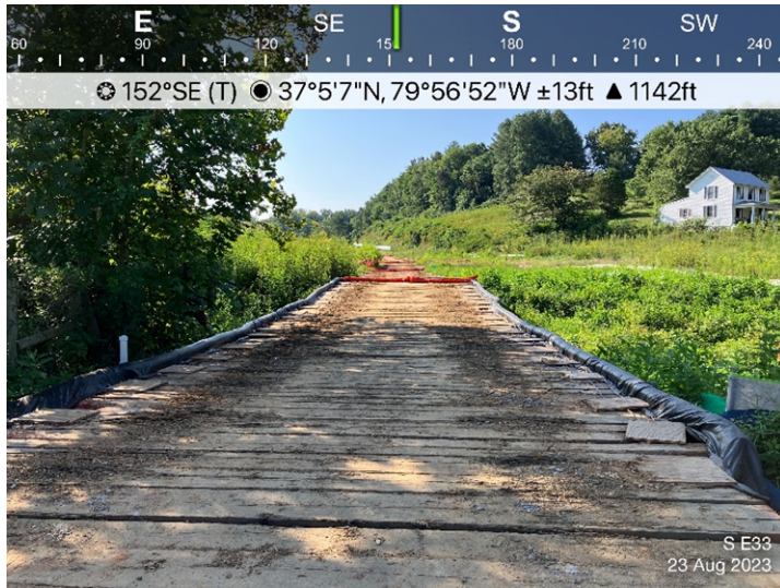
Figure 1: Designated crossing S-E33, ECD's are in place.
