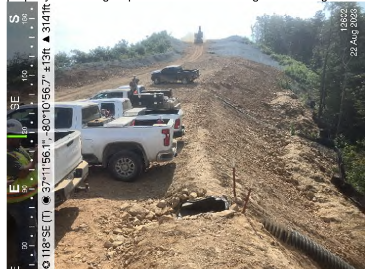
Figure 4: STA 12602+00 – Controls in place and functioning properly. Installing slope drains and stabilizing with matting.
