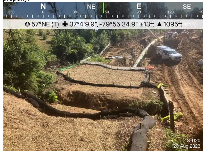
Figure 1: Stream S-D20 – Controls in place and functioning properly.
