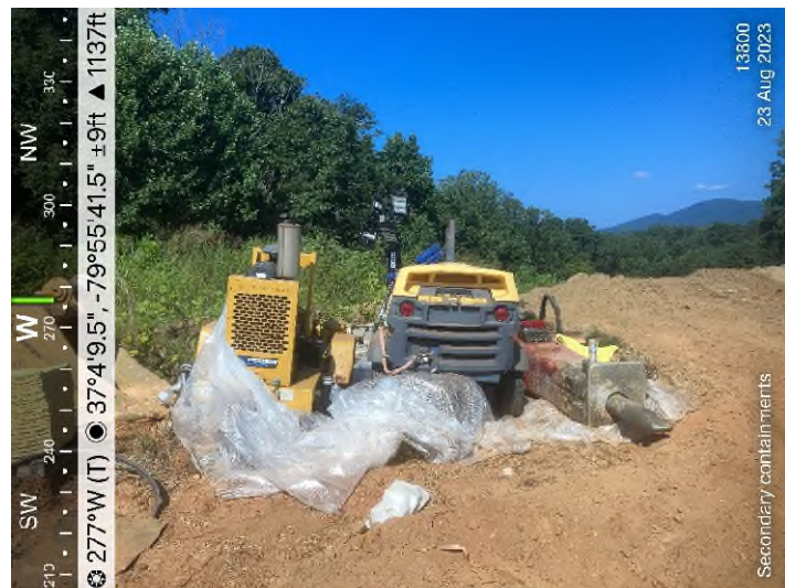
Figure 3: STA 13800+00 – install proper secondary containment.
