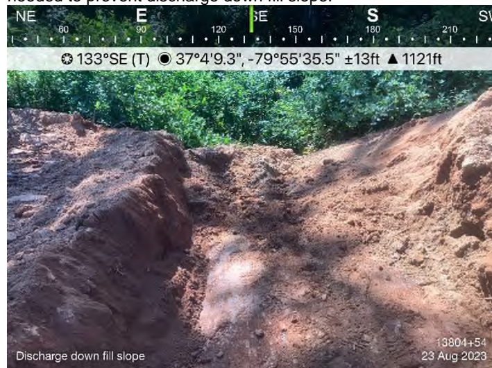
Figure 2: STA 13804+54 – Water bar flow path maintenance needed to prevent discharge down fill slope.
