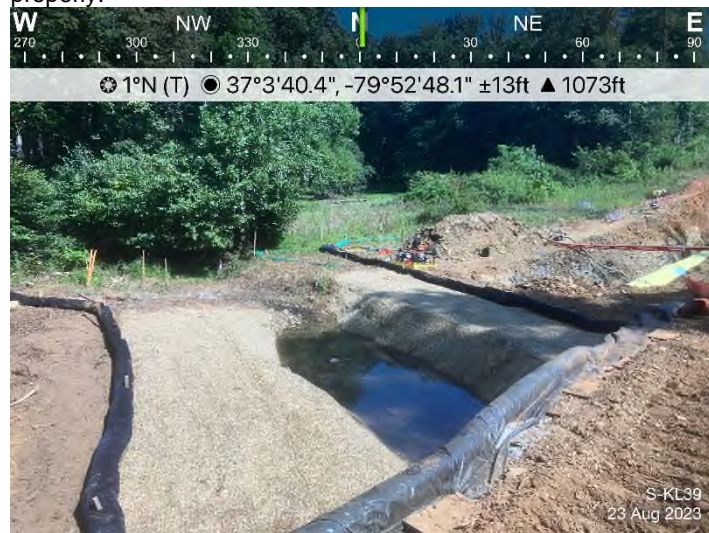
Figure 4: Stream S-KL39 – Controls in place and functioning properly.
