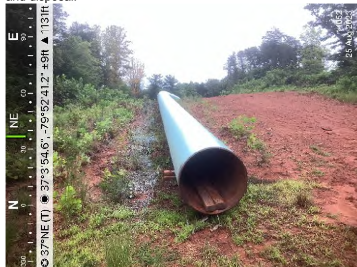
Figure 6: STA 14053+00 – Remove and properly dispose of over-sprayed vegetation. Ensure proper pipe remediation containment and disposal.
