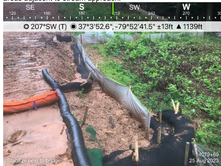
Figure 3: STA 14049+69 – Maintain CFS and stabilize disturbed areas adjacent to stream approach.
