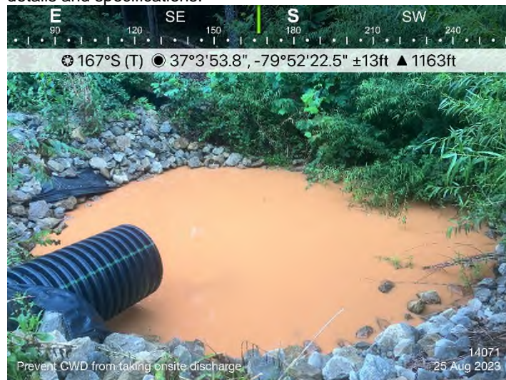
Figure 11: STA 14071+00 – Prevent onsite discharge from entering CWD plunge pool. Repair CWD as needed per approved details and specifications.
