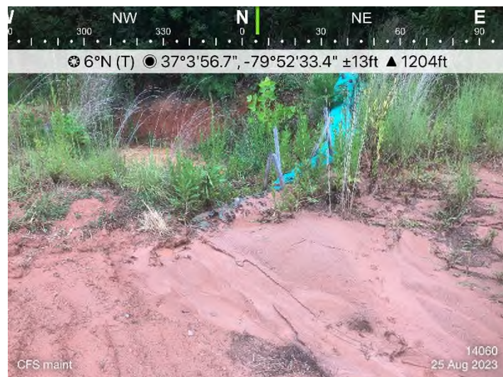
Figure 8: STA 14060+00 – Maintain/clean out CFS.
