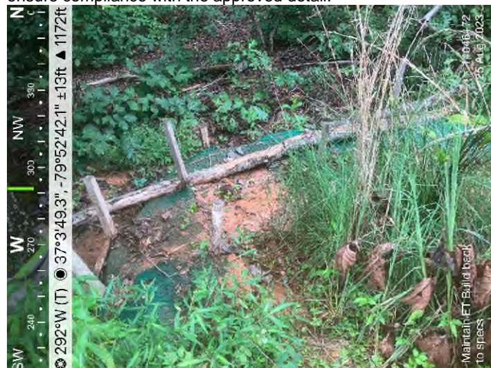
Figure 1: STA 14045+00 – Cleanout CFS and repair ET to ensure compliance with the approved detail.
