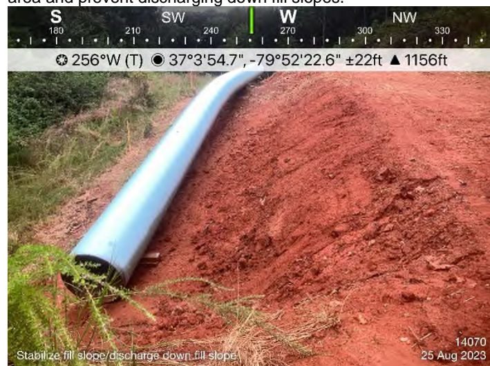
Figure 10: STA 14070+00 – Properly stabilize fill slopes in this area and prevent discharging down fill slopes.
